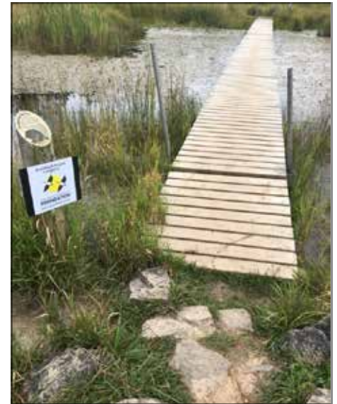
Boardwalk repairs at Bognor Marsh make for a sturdy hiking surface
